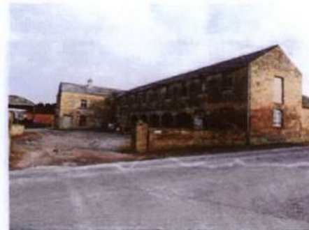
Estate Buildings at Birdsall
